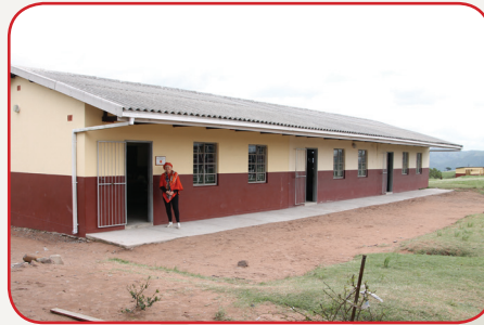
Construction of a Skill Centre
